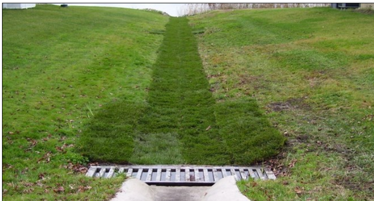
A bioswale is a stormwater best management practice.
